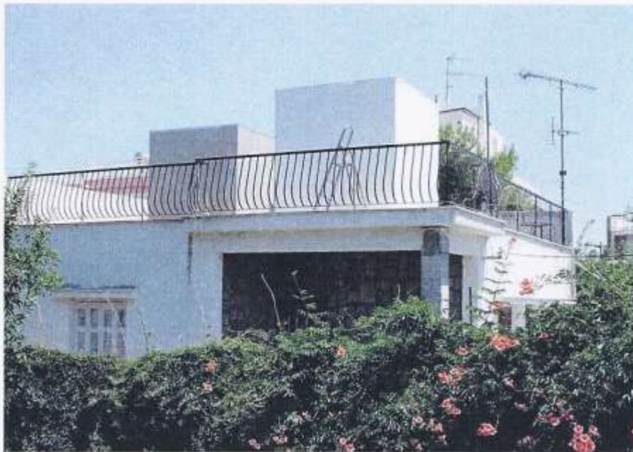
Figure 2. The two test rooms positioned on the roof – View from the West.
