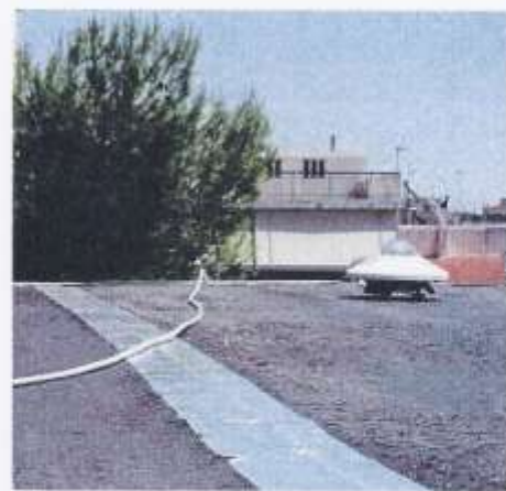
Figure 12. Solar radiation sensor on top of Test room 2 roof.
