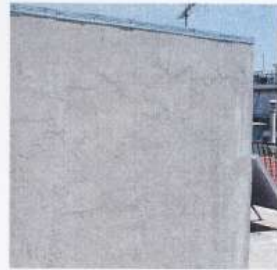
Figure 14. Test Room 2 - South wall.
